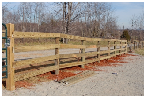
Picture 1 – Horizontal wood barriers
